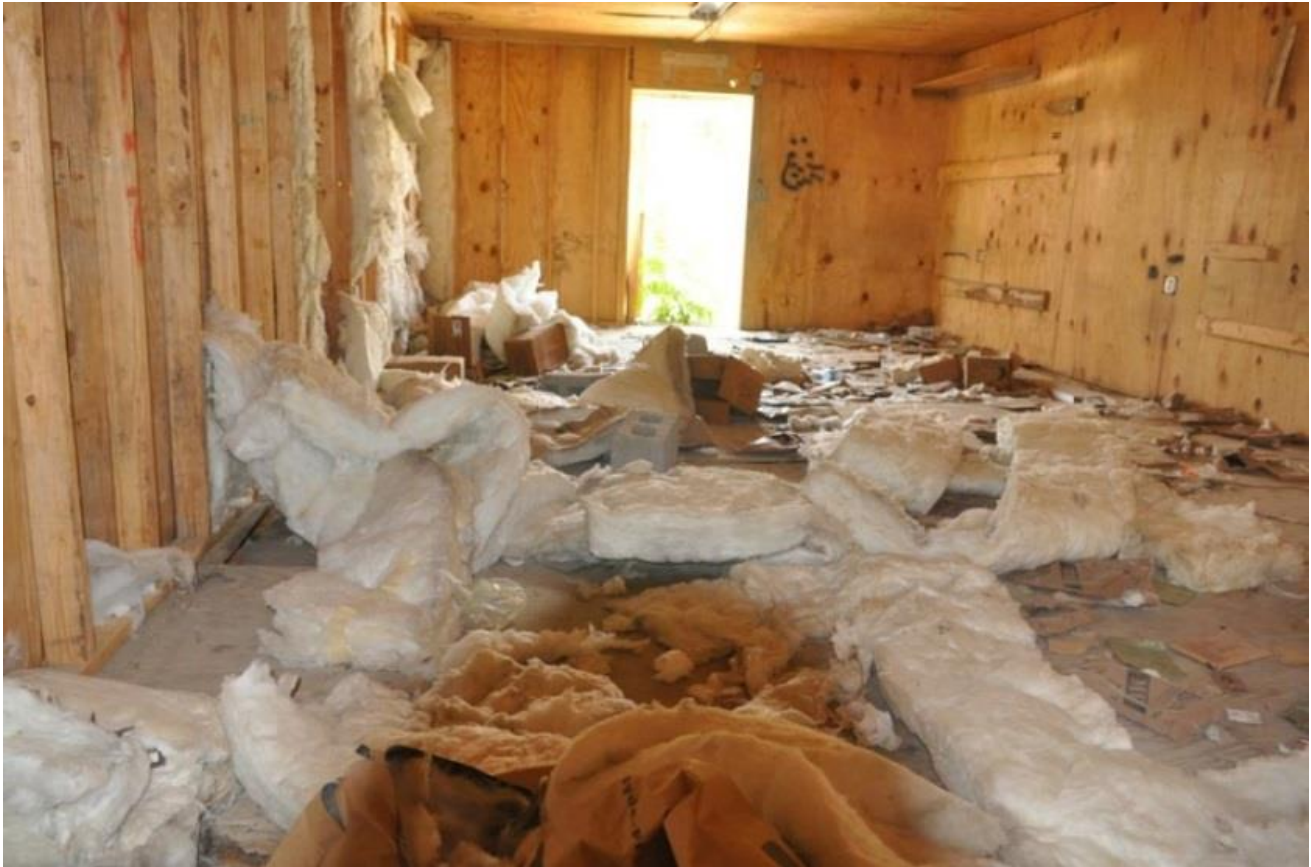
Several buildings at Nangalam Base, known as Forward Operating Base Blessing until the U.S. Army turned it over to Afghan forces in February, show signs of neglect. U.S. soldiers began moving back into the base in the Pech Valley of Kunar province in late July. MARTIN KUZ/STARS AND STRIPES
