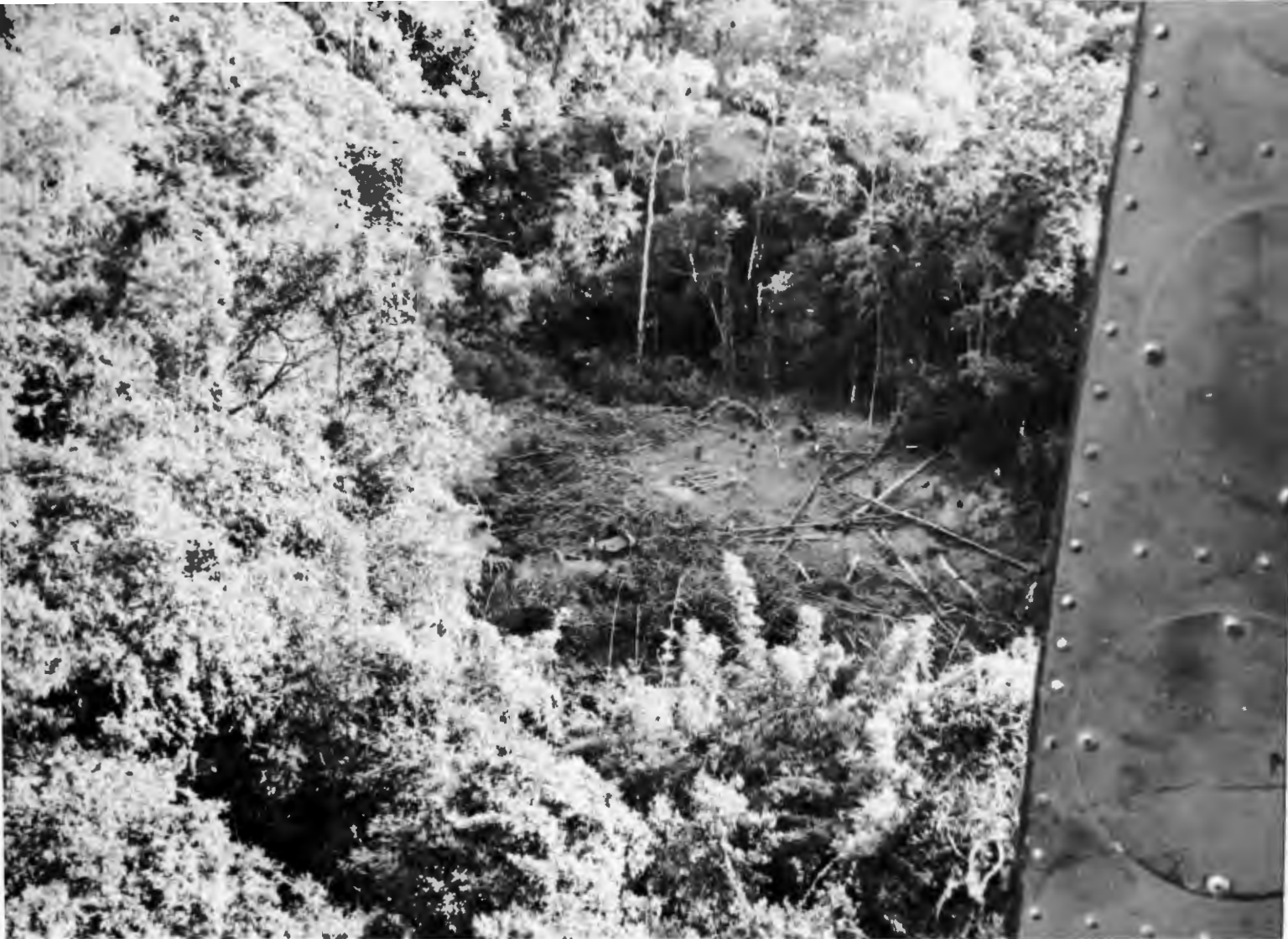
AERIAL VIEW OF LZ BEING CLEARED
