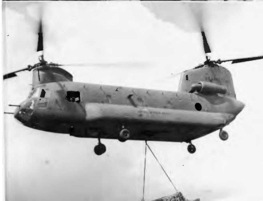
BRIDGE SECTION IS LIFTED BY "CHINOOK" HELICOPTER TO BRIDGE SITE
