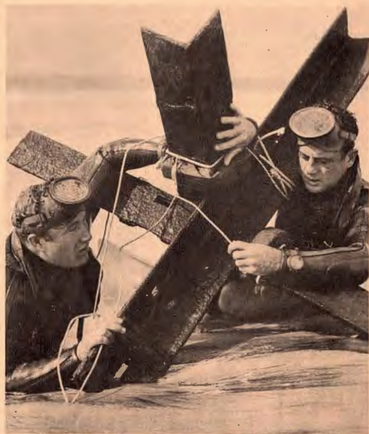
FROGMEN - Navy frogmen from an underwater demolition unit set demolition charges on a "hedgehog," a beach obstacle placed by the enemy to block entry to certain sections of the beach and to channel landings into areas which are heavily covered by pre-registered supporting arms. The highly trained and skilled frogmen also perform beach reconnaissance, mine field clearance, explosive ordnance disposal, inland demolition raids, salvage and sneak attacks.
